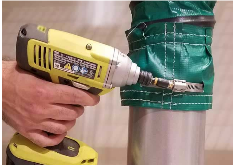
Figure 5 – Installing Flex-Duct on Tube
