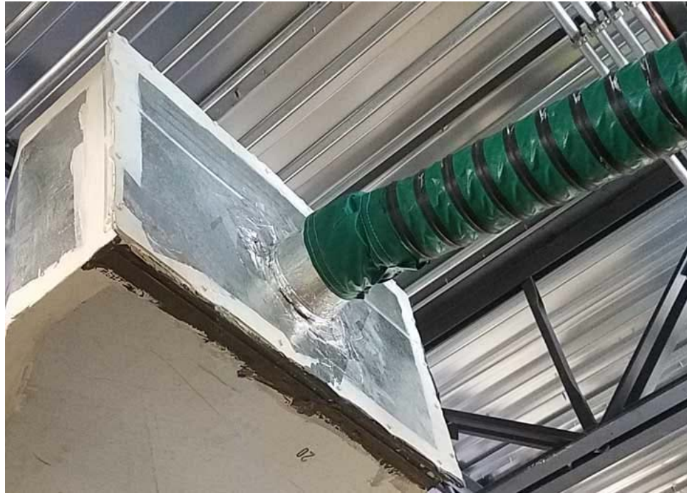
Figure 6 – Flex-duct Connection to Duct System
