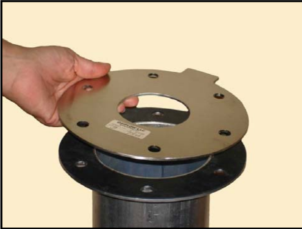
Figure 1 – Installing Orifice Plate
