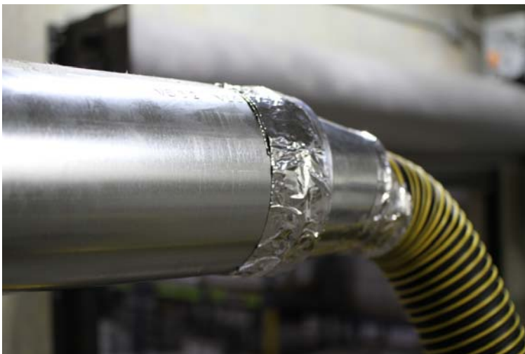
Figure 6 – Connection to Duct System
